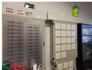
Graphic Annunciator Fire Alarm System
