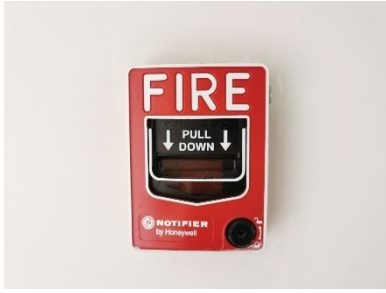
Fire Alarm Manual Station
